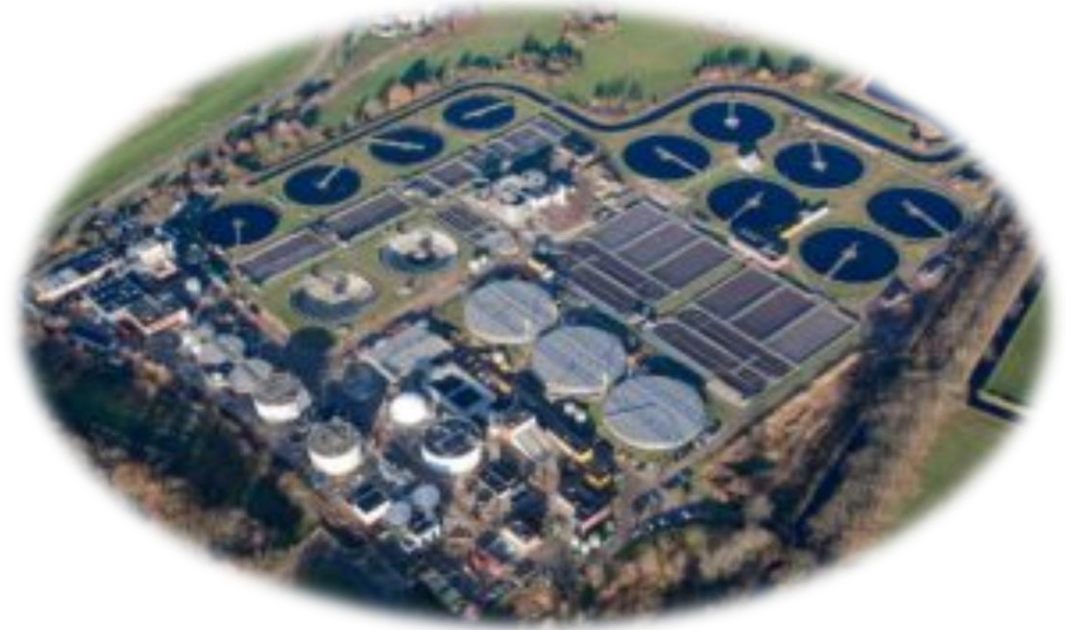
Aerial view of DARROW WWTP (Tilburg, Netherlands)
