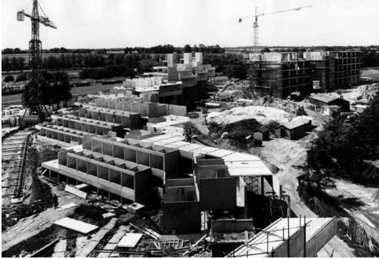
Fig. 4. The students residences under construction. Photo: Leigh, ARUP private archive.
