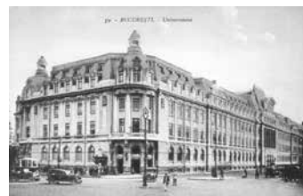
Fig. 1. University of Bucharest. The main part of the university was constructed in the 19th century. The building was expanded in the 1920s, with new wings added. Postcard, c. 1930s.
