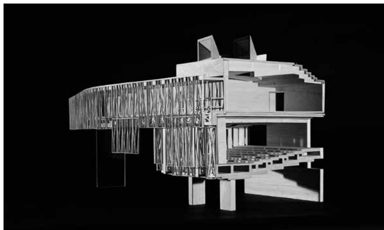
Fig. 6. Maquette of the main façade, composed of large steel portals containing scraps of Murano glass. Courtesy of Miralles Tagliabue – EMBT Architects. Photo by Lourdes Jansana.
