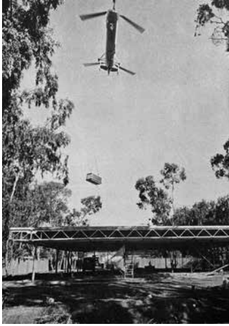
Fig. 4. A helicopter places the air-conditioning unit on the roof of Phase Two Mock-Up. SCSD, SCSD: An Interim Report , Educational Facilities Laboratories, New York (NY), 1964, p. 23.
