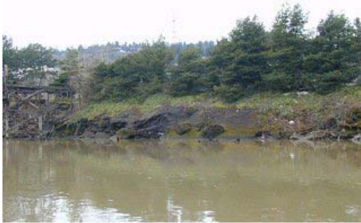
Asphalt slurry applied for river bank stabilization
