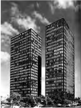
Lake Shore Drive. Chicago. Mies van der Rohe.
